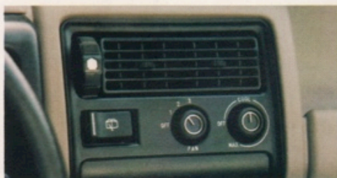
Le Car air conditioning
