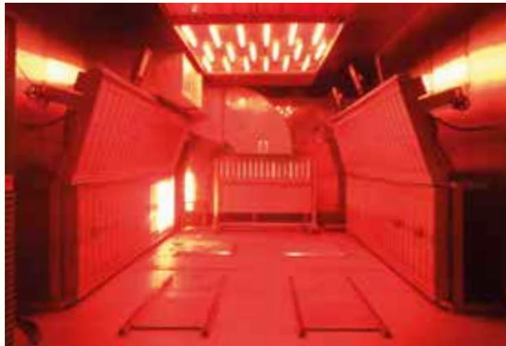
Honda climate chamber at our Swindon manufacturing facility.
